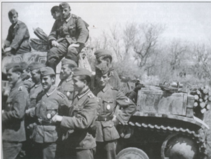
Several Pz.Kpfw.IIs, backed up by a Pz.Kpfw.IV, have halted for a maintenance break. Note that the nearest leichte Panzer (an Ausf.A, B or C) has the Vorpanzer (spaced armor) on the bow and Zusatzpanzerung (appliqué armor) on the turret front and superstructure, but retains the original split hatch lids on the turret roof. It wears a white two-digit Tac number, 31, on the turret side as well as a black/white Balkenkreuz on the superstructure side plate. Finally, it has lost the rod antenna storage trough normally seen mounted to the port side track-guard.
