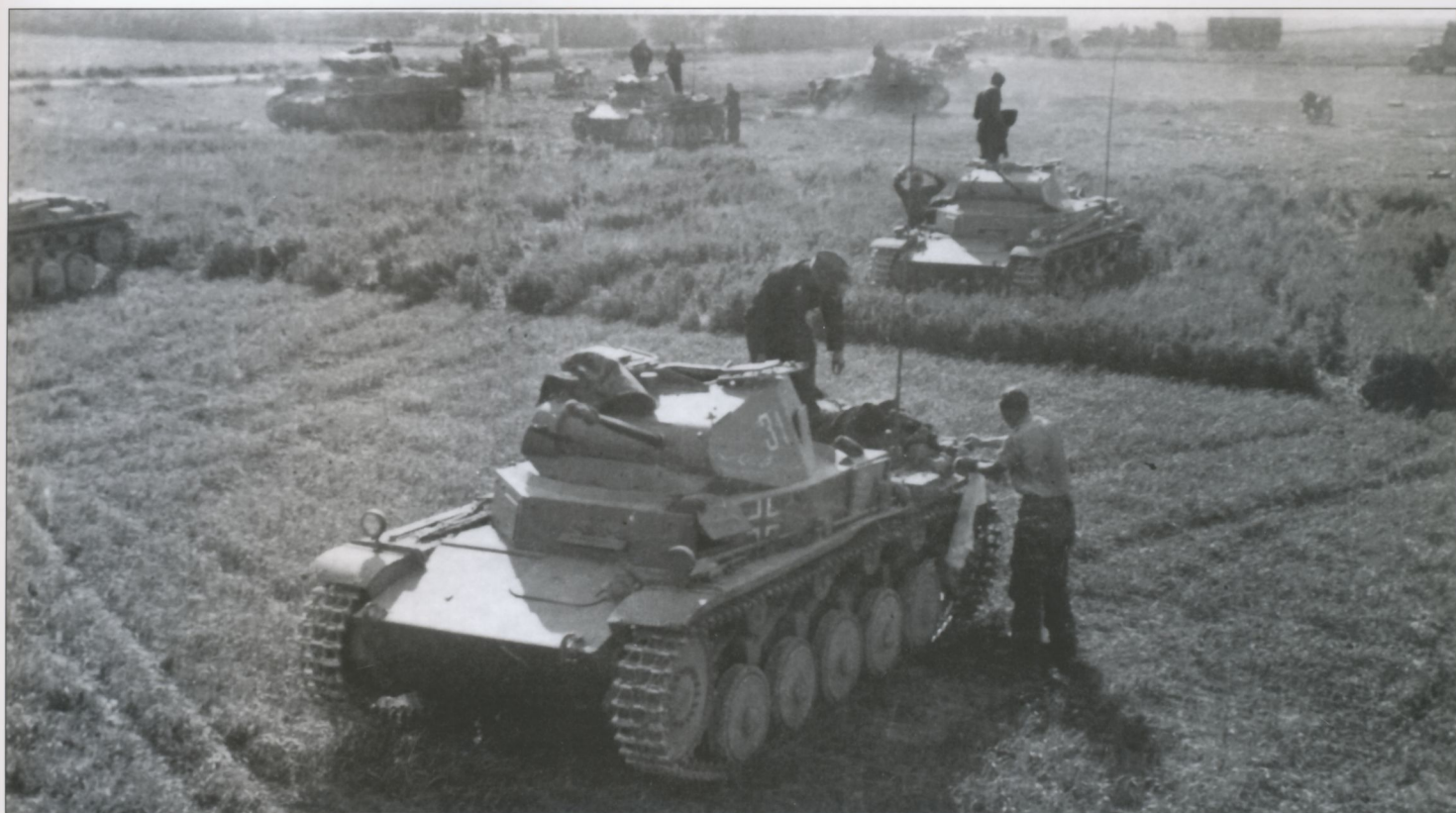
Several Pz.Kpfw.IIs, backed up by a Pz.Kpfw.IV, have halted for a maintenance break. Note that the nearest leichte Panzer (an Ausf.A, B or C) has the Vorpanzer (spaced armor) on the bow and Zusatzpanzerung (appliqué armor) on the turret front and superstructure, but retains the original split hatch lids on the turret roof. It wears a white two-digit Tac number, 31, on the turret side as well as a black/white Balkenkreuz on the superstructure side plate. Finally, it has lost the rod antenna storage trough normally seen mounted to the port side track-guard.
