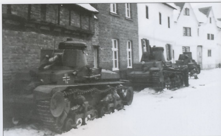
Prior to the French Campaign of 1940, Pz.Kpfw.35(t)s (as they were now designated) had their Balkenkreuz national insignia changed to a style that featured a thin white outline with a black core. Their position was also changed to three places on the hull/superstructure, instead of the previous four places on the turret. This pair of Panzer belonging to 6.Panzer-Division, are parked on the side of a street next to some local structures, during winter exercises.
