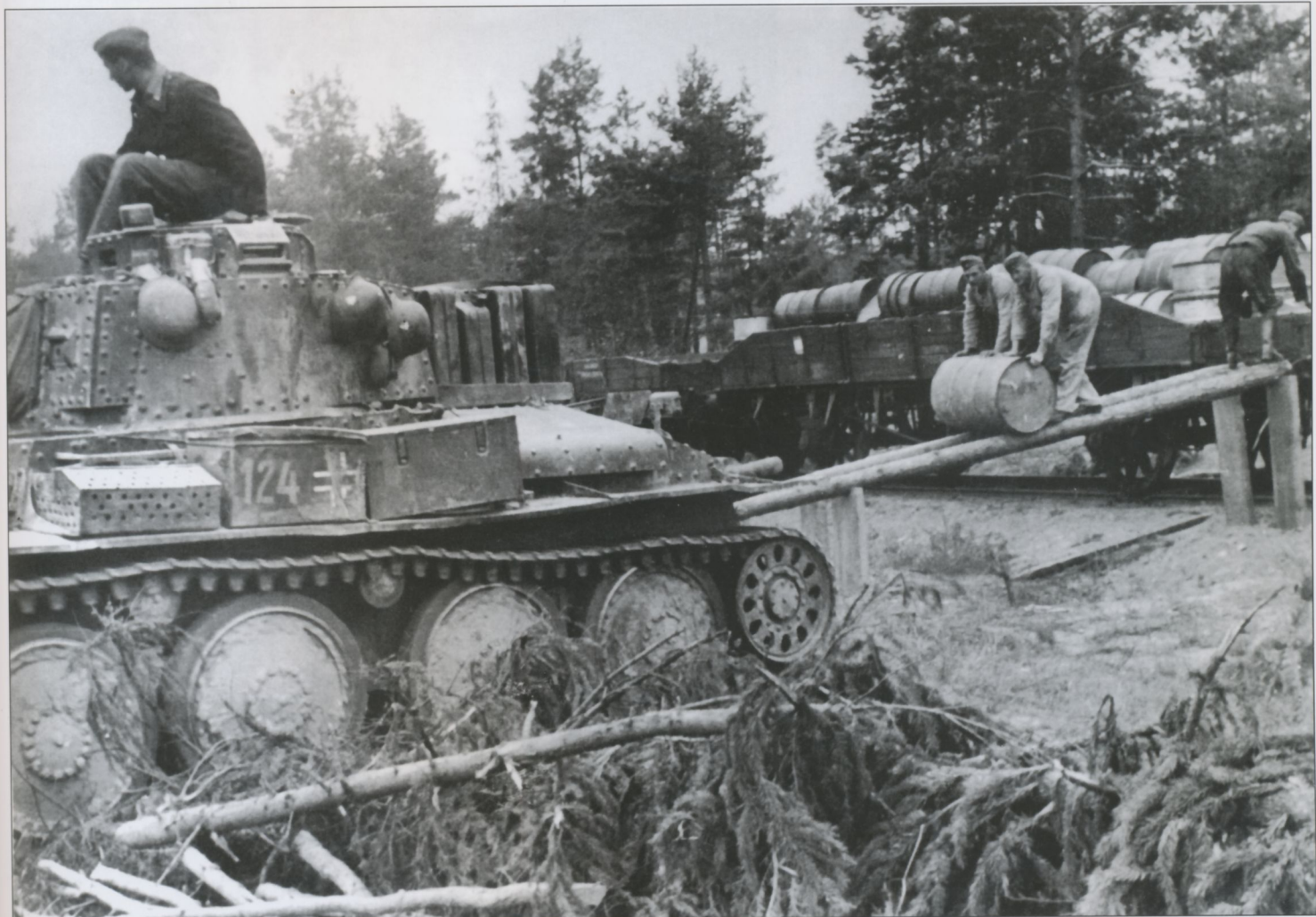
Sited next to a rail-head, this Pz.Kpfw.38(t) Ausf. B, C or D (identified by the bolt pattern on the turret front plate for 25mm armor) is either awaiting fuel or providing site security somewhere on the Ostfront, probably in 1942. Its stowage and markings pattern resemble that seen on Panzer of 12.Panzer-Division, while the crew has also stowed their water bottles on the turret exterior. A tray for 20-liter jerrycans is fitted to the engine deck; this was first seen during the French Campaign of 1940.
