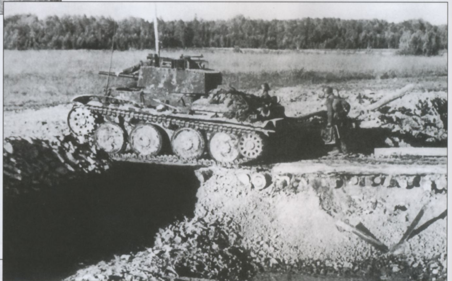
This Pz.Kpfw.38(t) Ausf. E, F or G is identified from this angle by the raised exhaust muffler, first introduced on the Ausf.E. Just below the muffler is the armored box containing a bank of Nebelkerzenabwurfvorrichtung (rack to deploy smoke candles). This image also affords an excellent insight into how German Pioniertuppen would prepare ditches for crossing by motorized transport and AFVs. Note the logs placed at right angles across the earth and stone road-bed; other logs are laid at a 90-degree angle atop them to provide a hard surface for vehicular traffic.
