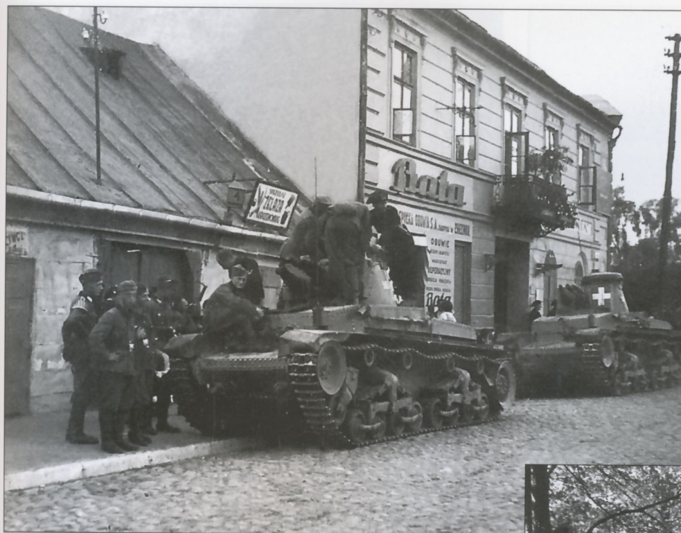
Parked on the side of a Polish street, one of a pair of Panzerkampfwagen (3.7cm) L.T.Sk.35s gets the "once-over" by a group of curious German troops. It is clearly seen how prominent the white Balkenkreuze national insignia were when viewed against the dark colors of the Panzer of the era. This led to over-painting in the field and a change to the insignia after the campaign's end.
