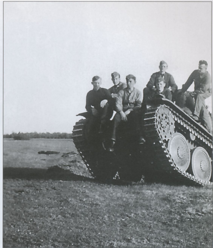
A Pz.Kpfw.38(t) of undetermined model is covered in troops, probably at a driver's training center. Note that the 3.7cm KwK(t) has not been fitted and that a Notek black-out driving head-lamp can be seen just over the front edge of the near-side track-guard. The lack of armament suggests that this is a Fahrschulepanzer.
