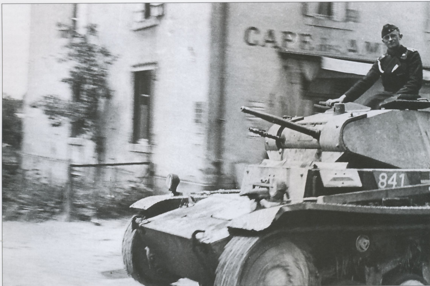
This photograph is unusual in that it shows the Notek black-out driving head-lamp mounted on the port side track-guard of a Pz.Kpfw.II Ausf.A, B or C obviously somewhere in France as denoted by the café sign on the building in the background. Whether this image was made during the actual campaign itself is open to conjecture since the leichte Panzer is devoid of any stowage on the usually cluttered bow. Note the Vorpanzer (spaced armor) on the bow and Zusatzpanzerung (appliqué armor) on the turret front and superstructure front; the commander's hatch lid is the original two-piece design.
