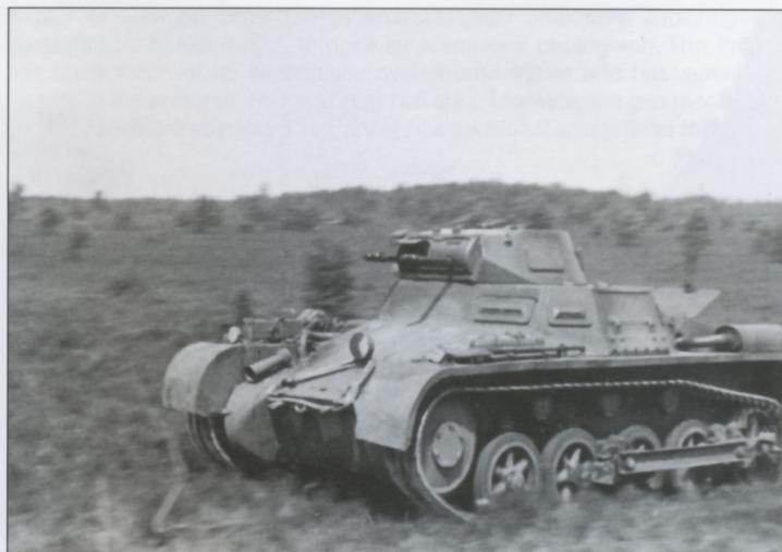
Moving at speed across a field, this Pz.Kpfw.I Ausf.A's tracks again display the illusion that there are no guide horns on the outside of the wheels. This very dusty Panzer has the visor above the starboard side MG13k flipped open and also has an access hatch lid on the engine deck propped in the open position. In both cases, having them open will improve cooling, but will also allow more dust to enter the interior than would normally be the case.
