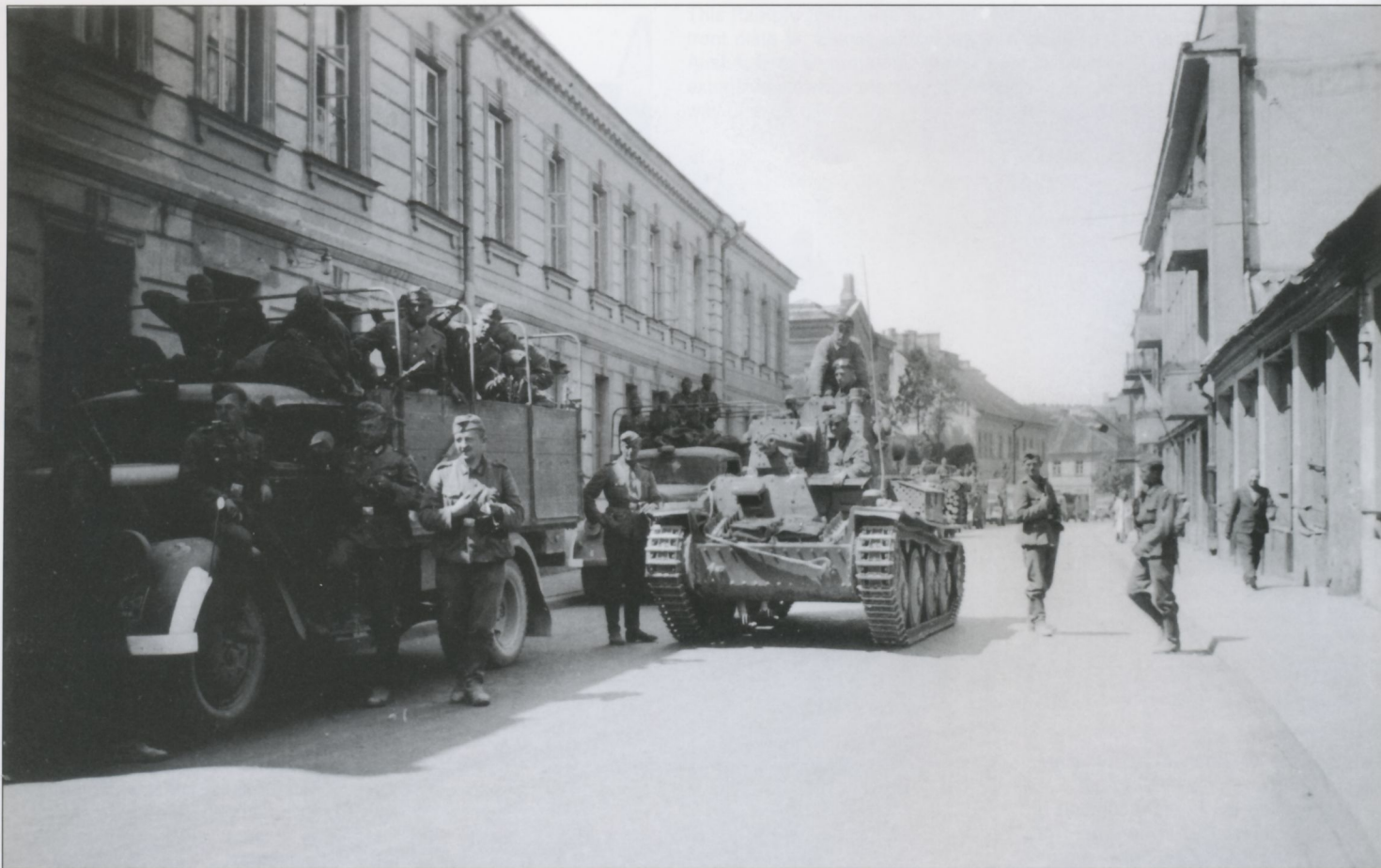
This Pz.Kpfw.38(t) Ausf.E or F als Zugfr.Wg (identified by the radio operator's visor and blanking plate over the former 7.92mm MG37(t) mount on the superstructure front plate) appears to be providing security for the pair of troop-laden Opel Blitz 3-ton trucks seen on the streets of a German-occupied city. Note the stowage locker (in this instance, the perforated front end is shown) and the bundle of wired-together saplings on the port side track-guard.
